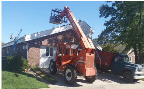
Roof Replacement - Summer 2014.
